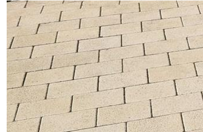
Front gardens sandstone paving
