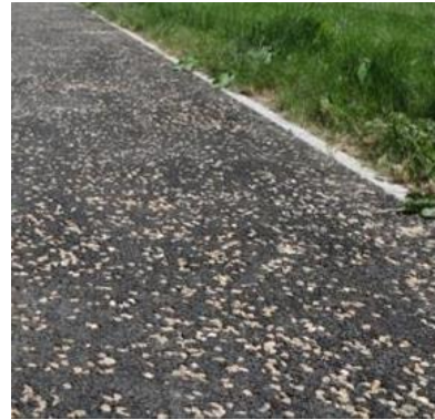
Hot rolled asphalt with variations in colour and texture provided by the inclusion of coloured aggregates or resin bonded surface finishes.
