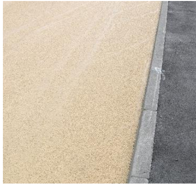
Hot rolled asphalt with variations in colour and texture provided by the inclusion of coloured aggregates or resin bonded surface finishes.
