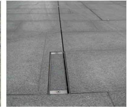
Recessed service covers and slot drains in plaza
